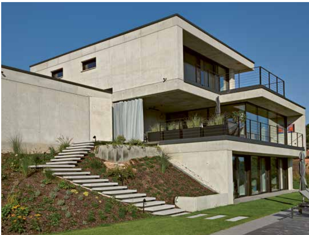
GDM.MASSIMO podest 150/50/8 cm, ferro soft, Staubgrau
